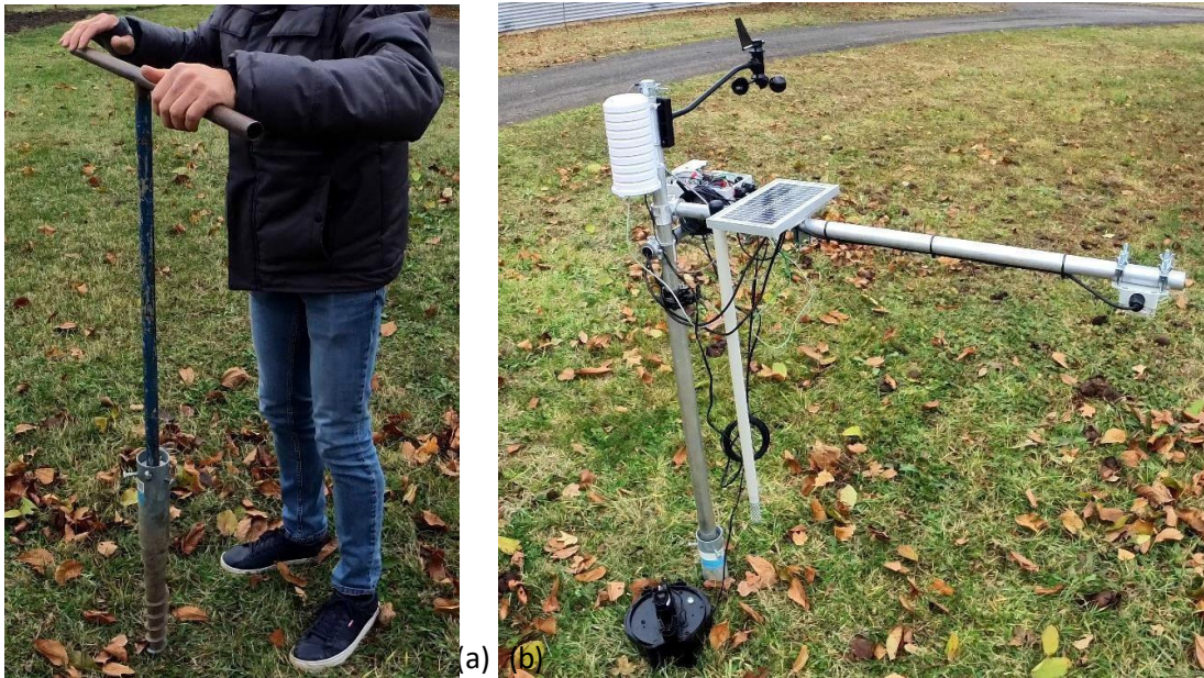
Figure 12. Major Step in Field Installation: Insertion of the screw-in stick that will secure the post in the ground (a) and fastening the post to the screw-in stick (b).
